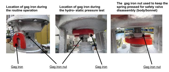
The gag iron shall be removed (located back to yoke extension piece) and the control unit shall be put into operation when the pressure test is finished.
