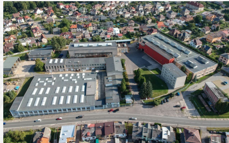
Production and administrative facilities of former Armaturka (Sigma), headquarters of LDM since 2002
