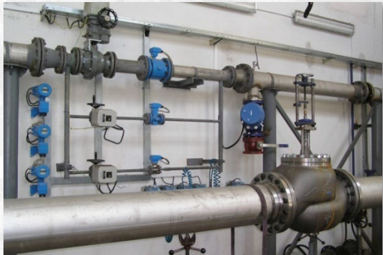
Testing of flow characteristics and Kv values
